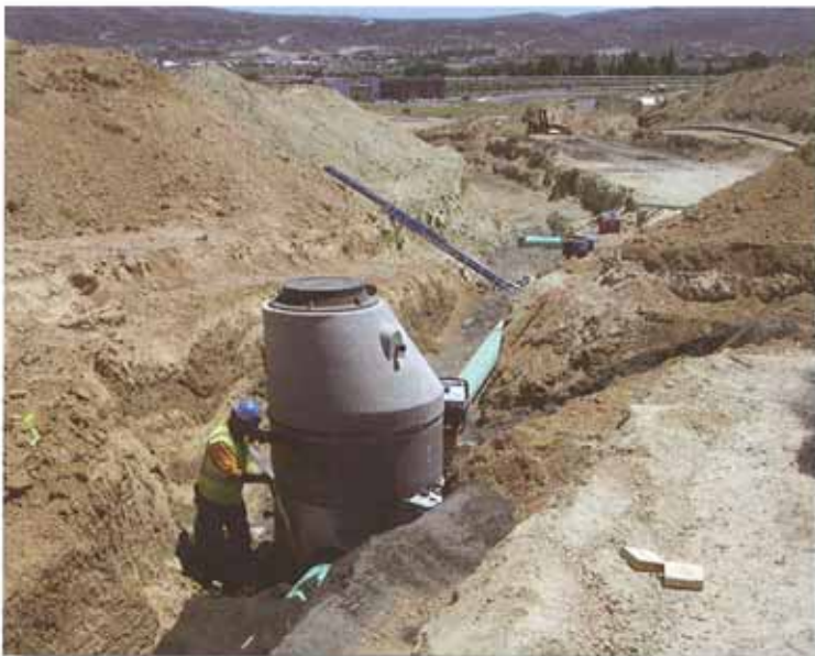
Installation of a sewer manhole.
