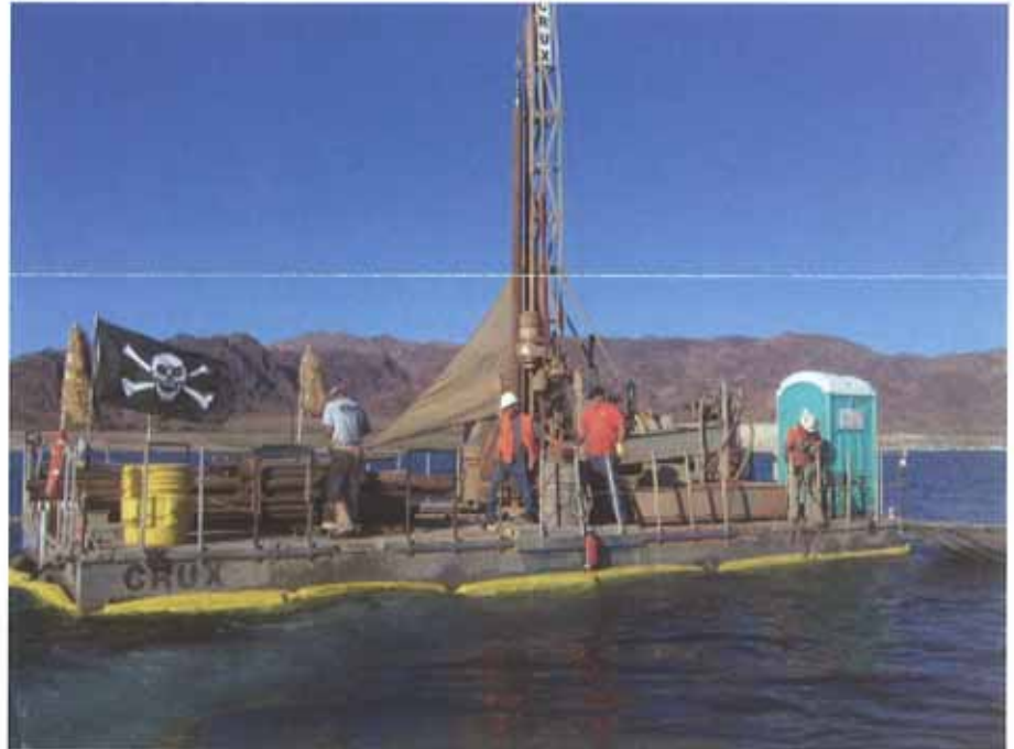
Barge Drilling with Crux Subsurface on Lake Mead
